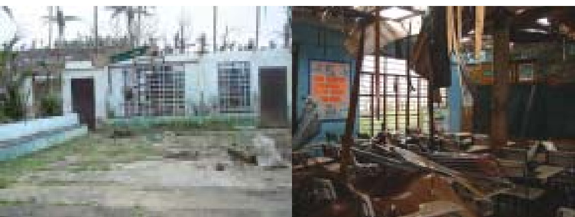
Damaged School Buildings
